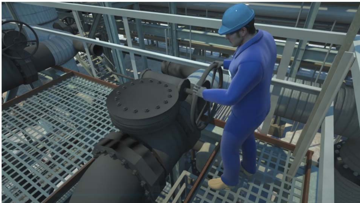
Figure 7. CSB Animation of Operator Opening Long-Winded Valve on Night of Incident. Valves on heat exchanger structure had to be opened concurrently when performing the heat exchanger bank startup
